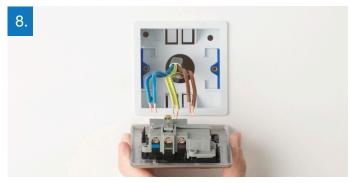
Line up the new socket and take note of where each terminal is located.
