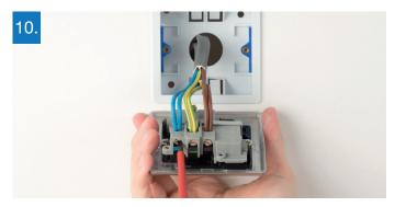
Make sure that the wires are fully inserted into the terminal and that no bare copper wire is visible. Tighten the screws securely onto the copper wire, not the outer sheeting.
