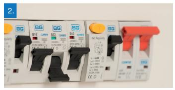
At the consumer unit, find the trip switch which protects the circuit and turn it all the way off. The indicator window should stay green.
