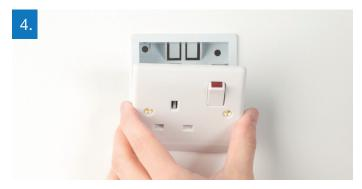
Gently ease the socket from the mounting box to show the wiring.
