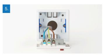
There will generally be three different wiring configurations. This photo shows a single wire of each colour connected to each terminal.
